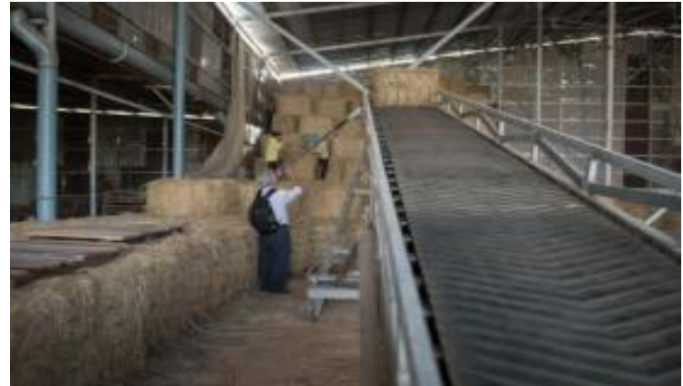
Straw warehouse (with conveying system)
